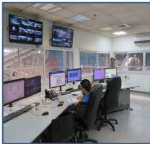
ELKAYAM Management and Control System.
